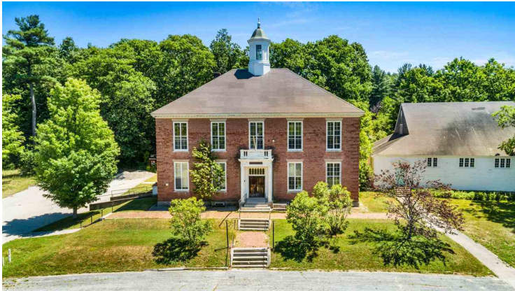
Figure 2 Appleton Academy Building, New Ipswich, NH
